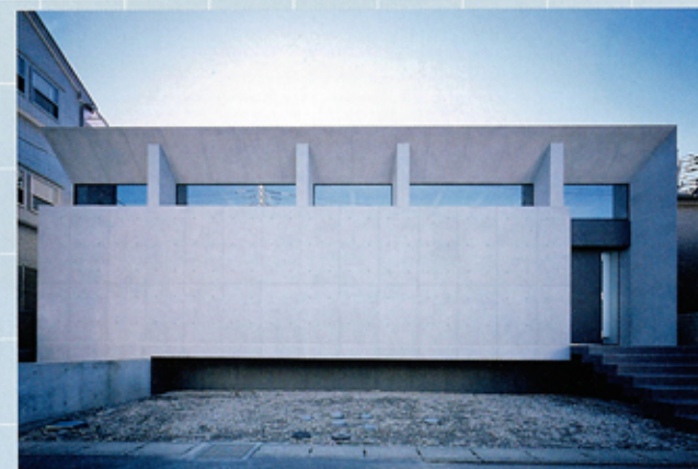
Photograph=西川公樹
